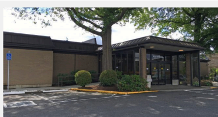
Providence Milwaukie Hospital (1 gallery) 10150 SE 32 Ave. Milwaukie
