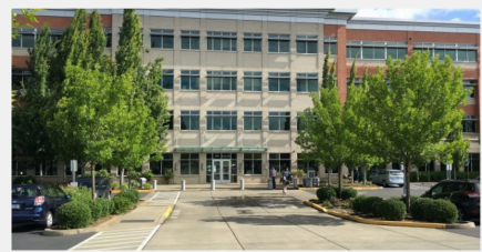
Clk Cty- Public Services Building Oregon City (3 galleries)
